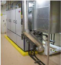
Figure 6a. CHP Unit (front and back views with heat recovery piping)
